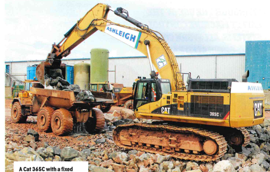
A Cat 365C with a fixed rock grab immediately loads the armour into the waiting fleet of Volvo ADTs.
