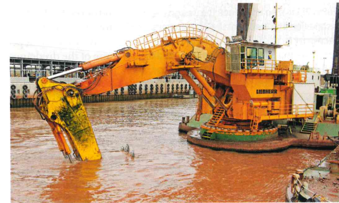
The dredged material was loaded on barges that made the short journey to the reclamation area, to be offloaded by a pontoon-mounted upper-structure of a Liebherr HS853 crane.
