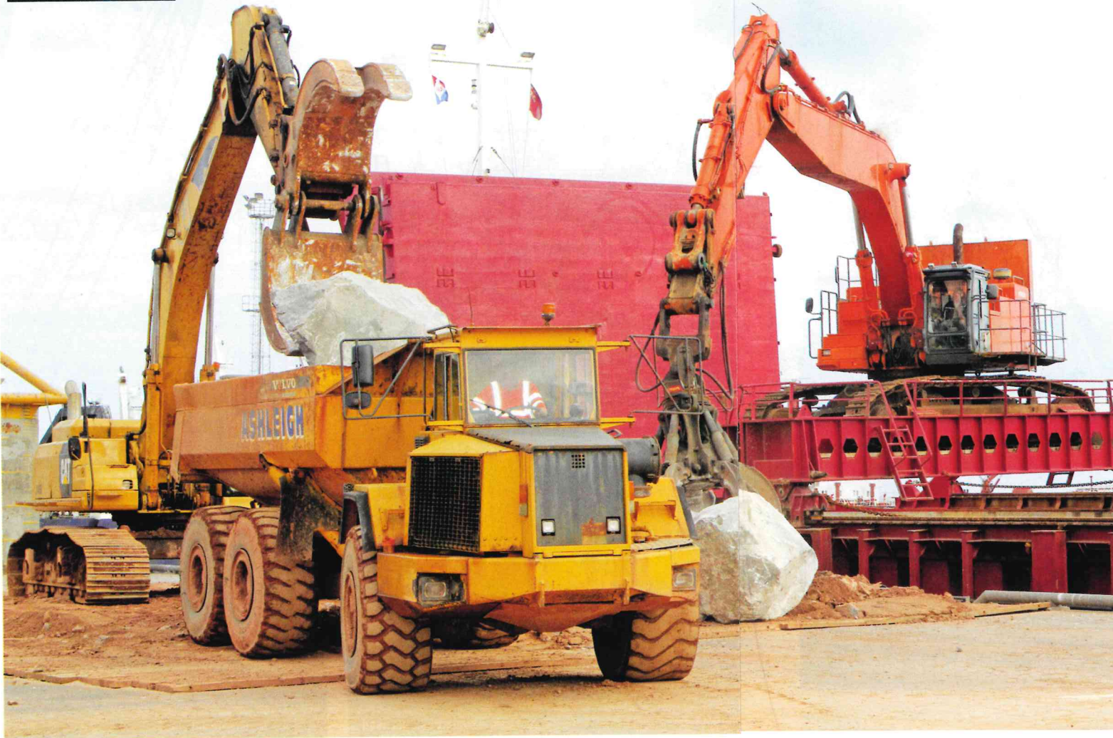
A Cat 365C with a fixed rock grab immediately loads the armour into the waiting fleet of Volvo ADTs.
