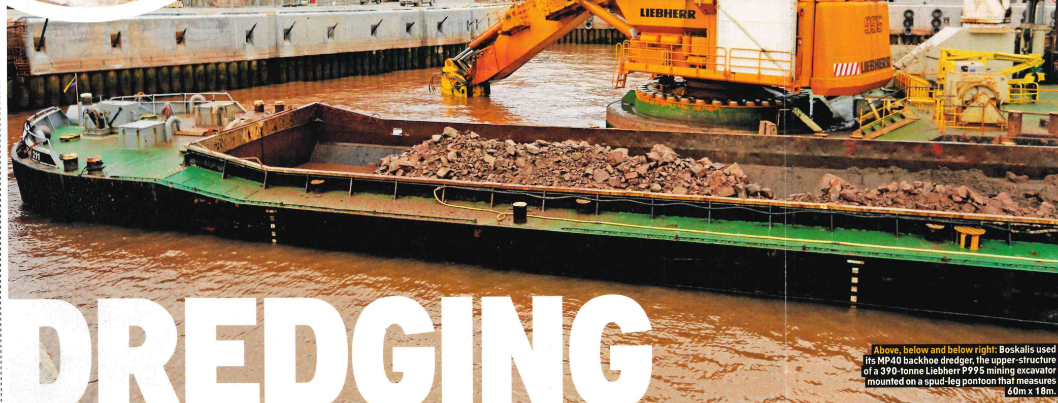
The dredged material was loaded on barges that made the short journey to the reclamation area, to be offloaded by a pontoon-mounted upper-structure of a Liebherr HS853 crane.
