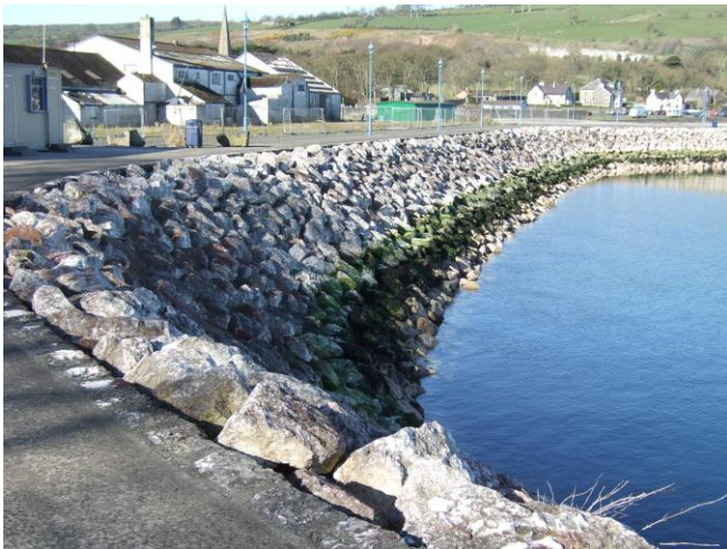
Inner Harbour protected with limestone armour
