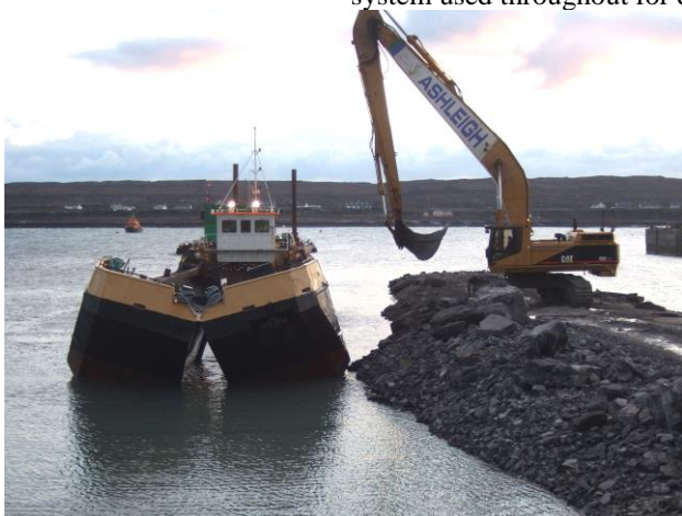
Views of dredging, sand retrieval, importation of Armour from mainland and Breakwater Construction
