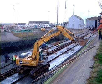
Preparation for and concreting of 150mm deep "overlay" slab over the existing slipway
