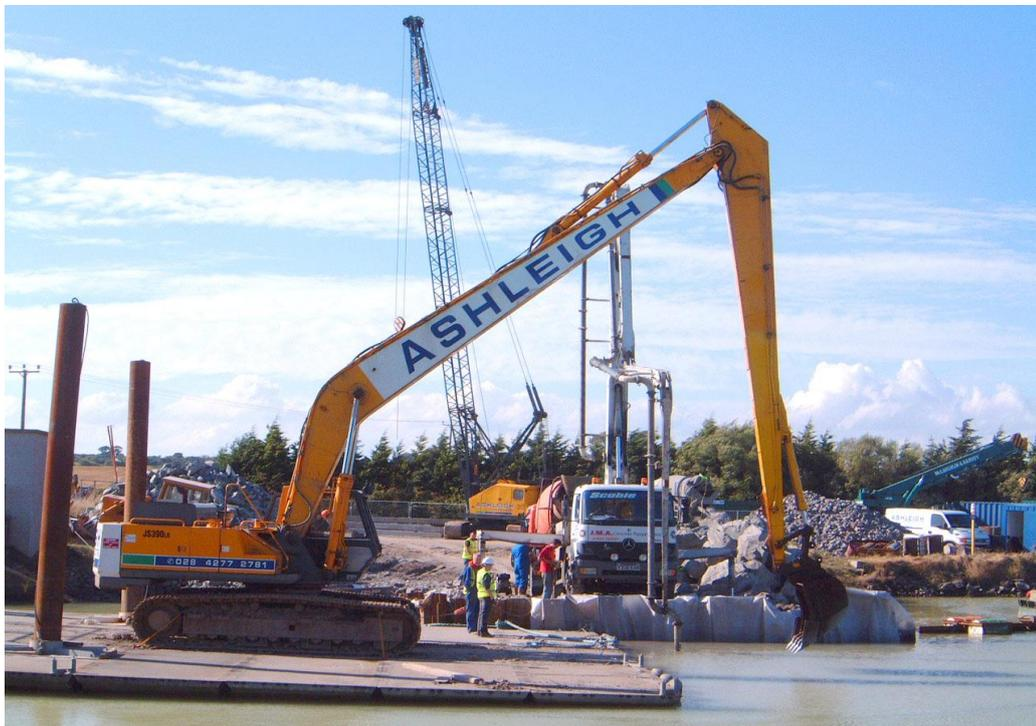
*Underwater concreting of scour protection apron using concrete pump with levels controlled by electronic "Digmaster" system fitted to 40T Long Reach excavator.*
