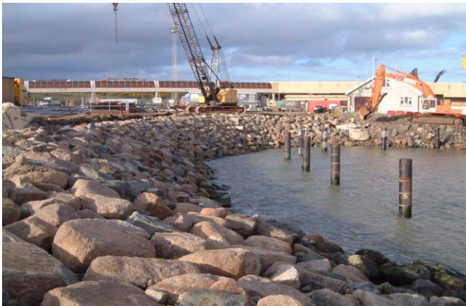
40T Long Reach Excavator with 19m Boom Length and 45T Excavator with underwater MSB800 Rockbreaker – during early stages of the formation of the new breakwater.
