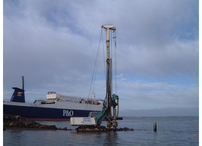
Drilling Rig installing 18m long Dia. 457mm piles through temporary filled piling platform for installation of piles 3m into bedrock
