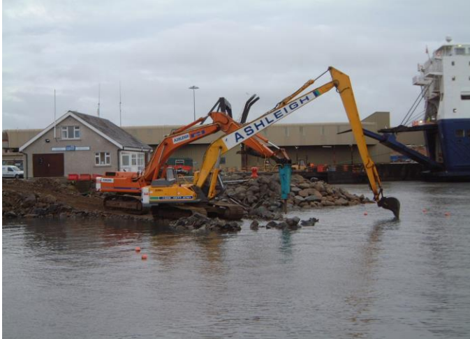
40T Long Reach Excavator with 19m Boom Length and 45T Excavator with underwater MSB800 Rockbreaker – during early stages of the formation of the new breakwater.
