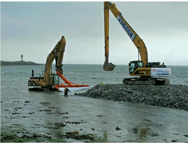
Excavation of Toe for North Revetment
