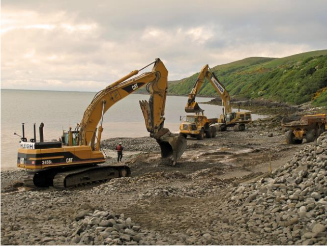
Excavation of Toe for North Revetment
