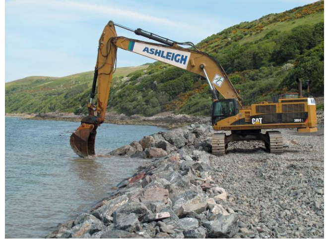
Construction of 2T to 4T North Revetment.
