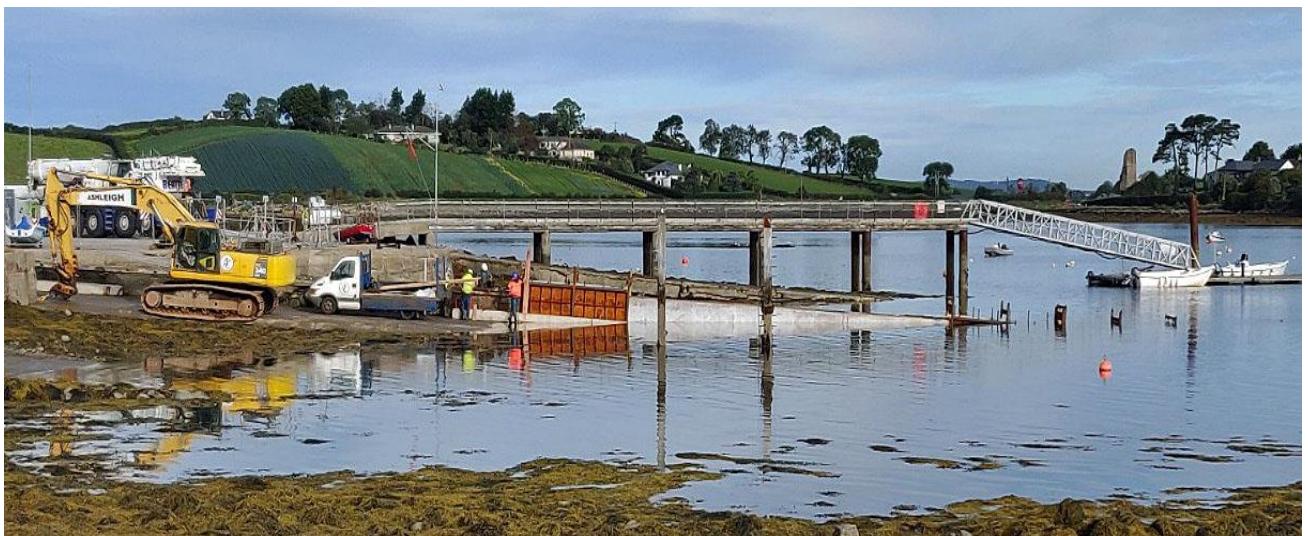
View of the Jetty encasement along the profile of Slipway No. 1
