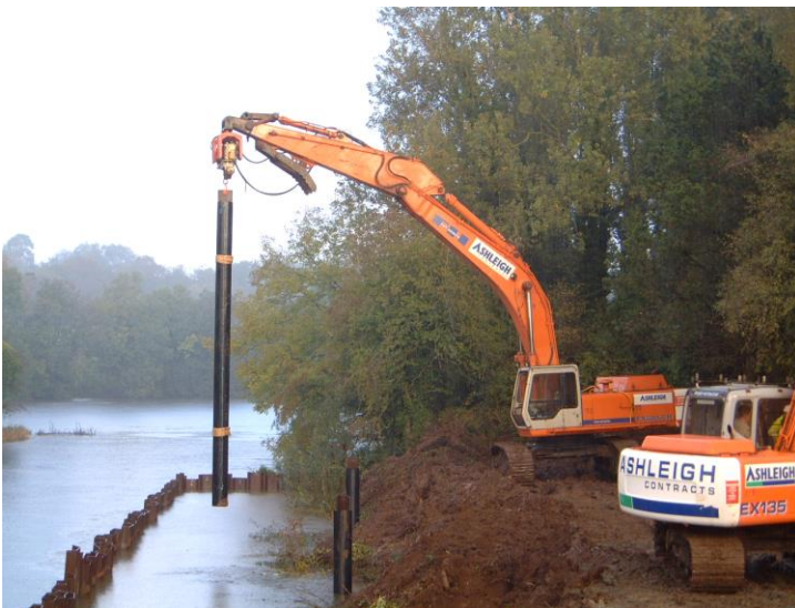
Excavator Mounted Vibrating (EMV400) Piling Hammer
