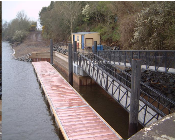
Completed jetty and pontoon at Carnroe.
